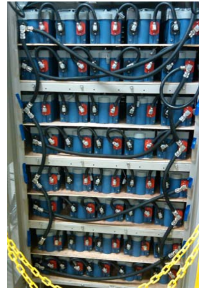
Figure 2. Ultracapacitor modules easily fit into standard UPS battery racks.
